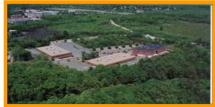
Corporate Headquarters, Manufacturing Milford, MA
